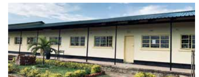
▲ Sino-Metals Leach Zambia Limited assists in the construction and renovation of the Zambian Chambishi Secondary School.
