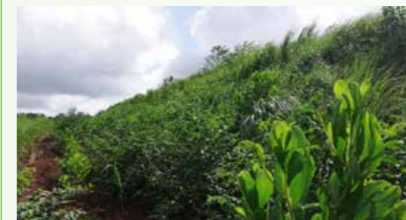
▲ Layered slope in the dumping yard of CNMC Nickel Co., Ltd.
