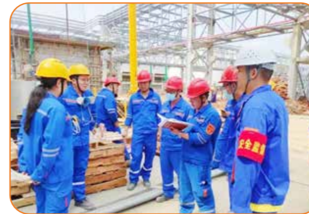
Hongsheng Copper carries out comprehensive inspections of safety, fire protection, and facilities.
