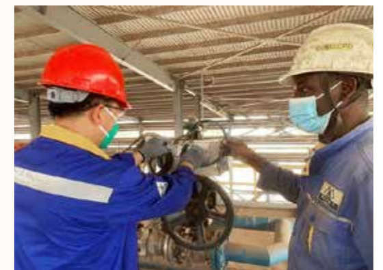
▲ Joint safety and quality inspections
